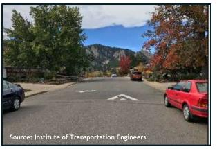
Speed bumps are additional asphalt with a substantial vertical deflection (i.e., a bump) installed across the width of the roadway that forces drivers to slow down to travel over. Speed bumps are generally installed in series along a roadway. Studies have shown that speed bumps installed at spacings of 260 to 600 feet provide optimal speed reduction along the length of a roadway.
